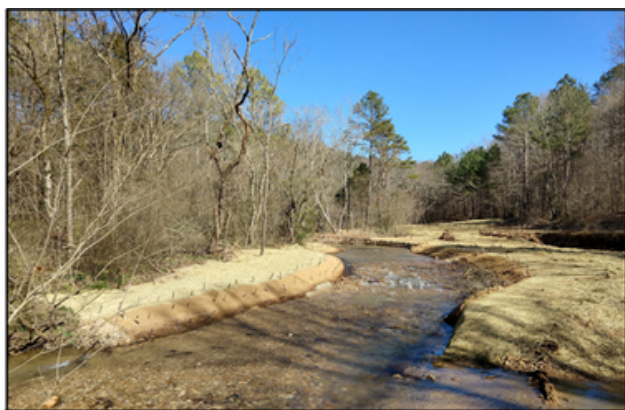
Loc. A, initial work (Feb 2022)
