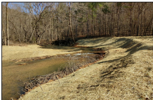
Loc. B, initial work (Feb 2022)
