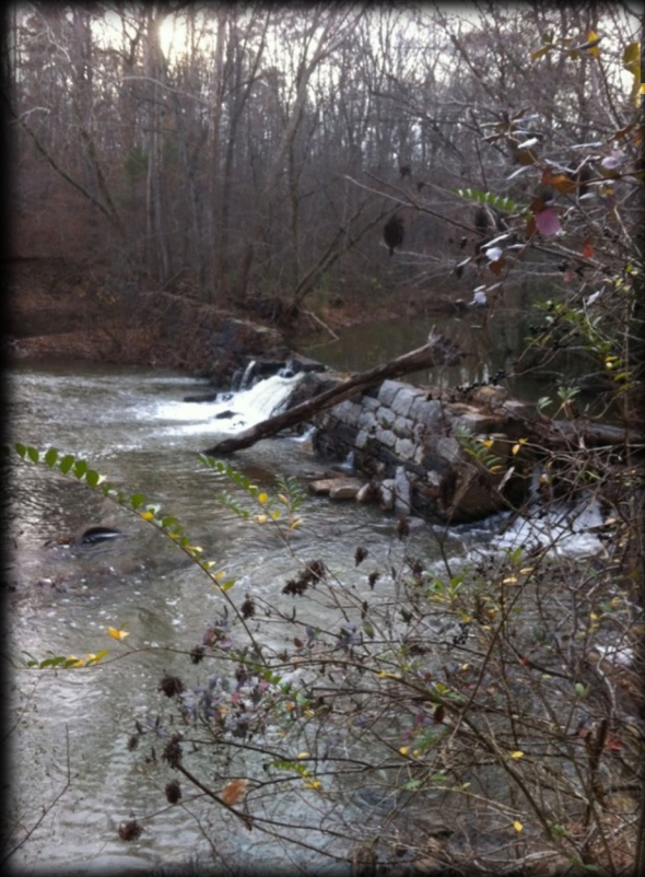
Pre dam removal
