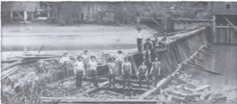
A photo of workers rebuilding Goodwin's Mill Dam, likely from the 1920s
