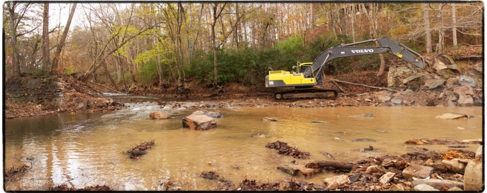
An excavator operated by U.S. Fish & Wildlife Service removes stones from the dam and uses them to restore stream bank
