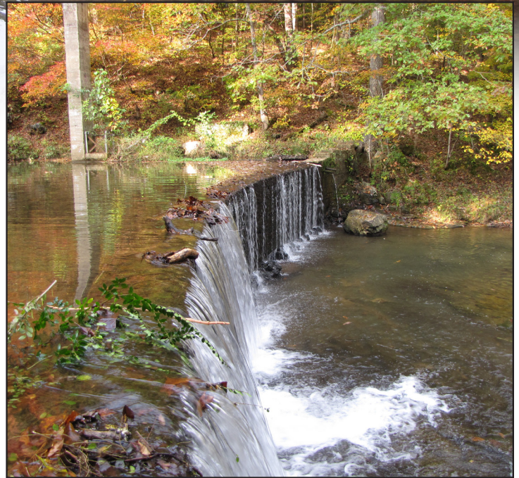
Old Shadow Lake Dam near Pinson AL
